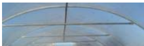
Crop support bars can be used to tie off plants and they also add 10% to the frame strength
